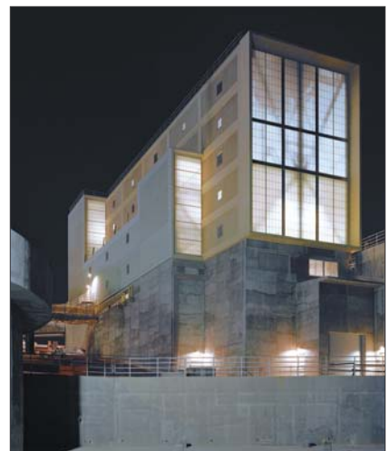
Translucent panels provided the opportunity to generate a soft glow from the center of the plant at night.
