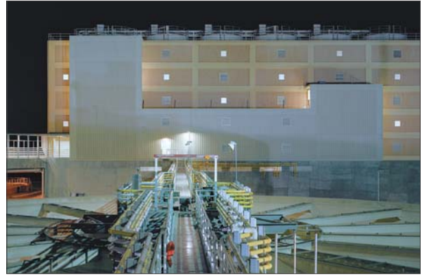
To reduce the impact of the largest building, lime silos were allowed to protrude beyond the roof.
