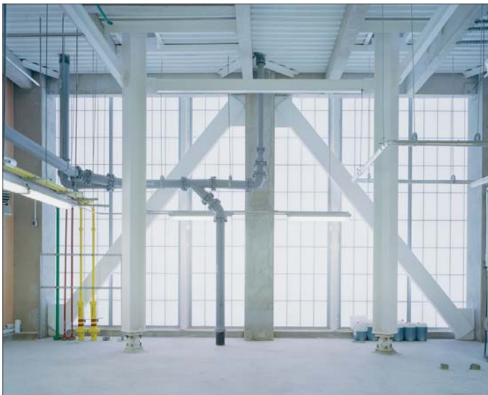
Interior daylight lighting at the Ullrich Water Treatment Plant.
