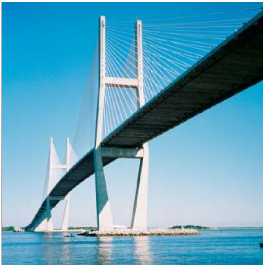
The bridge foundations are performing well under the loads of the completed bridge.
