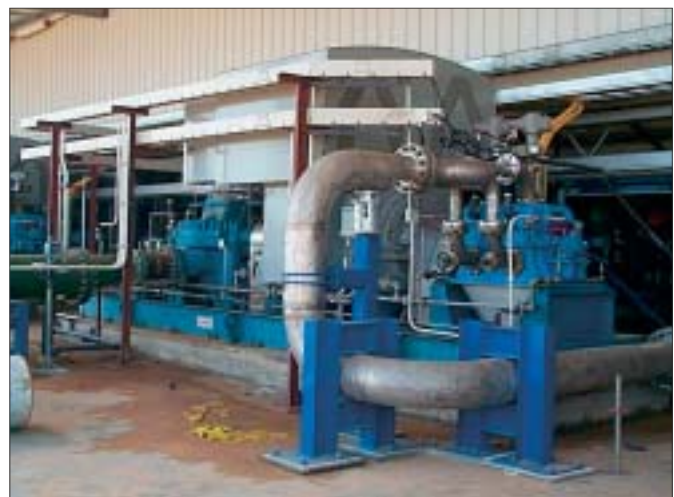
Largest Pelton Wheel energy recovery system in the world in Trinidad.
