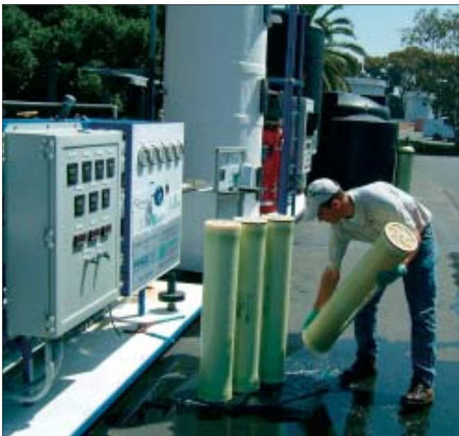
Reverse osmosis membranes—the work horses of today's desalination plants.
