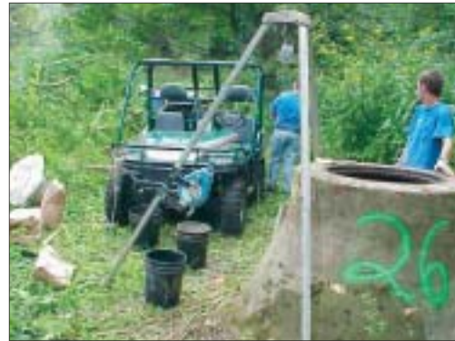
All-terrain vehicles transport materials and lightweight equipment to the more remote locations of Lowries Run.
