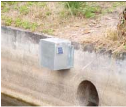
Solar-powered automated herbicide pellet distributors control floating vegetation within the 12 drainage basins located in Orange County.
