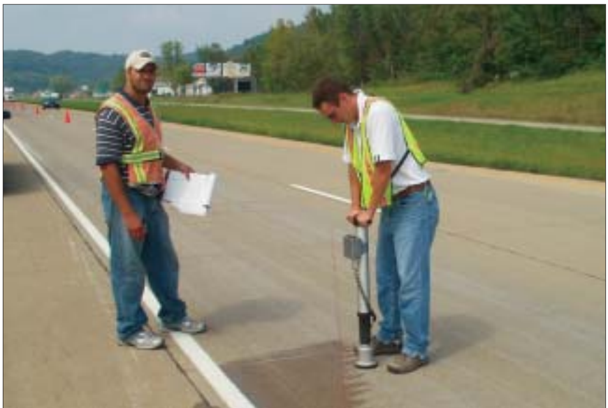
ORITE research personnel reading road salt residue levels using a modified Boschung SOBO-20. The white lines in the traffic lane are where the streams of brine were deposited.
