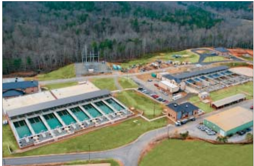
To avoid service interruptions while expanding the treatment capacity of its Etowah River Water Treatment Plant, the Cherokee County Water and Sewerage Authority built a new drinking water facility, shown at left in this photo, parallel to its existing facility, shown at right, which is being upgraded.
