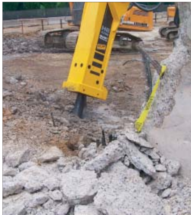
The AutoControl system allows the breaker to sense when the material is solid before allowing it to work at 100 percent capacity.
