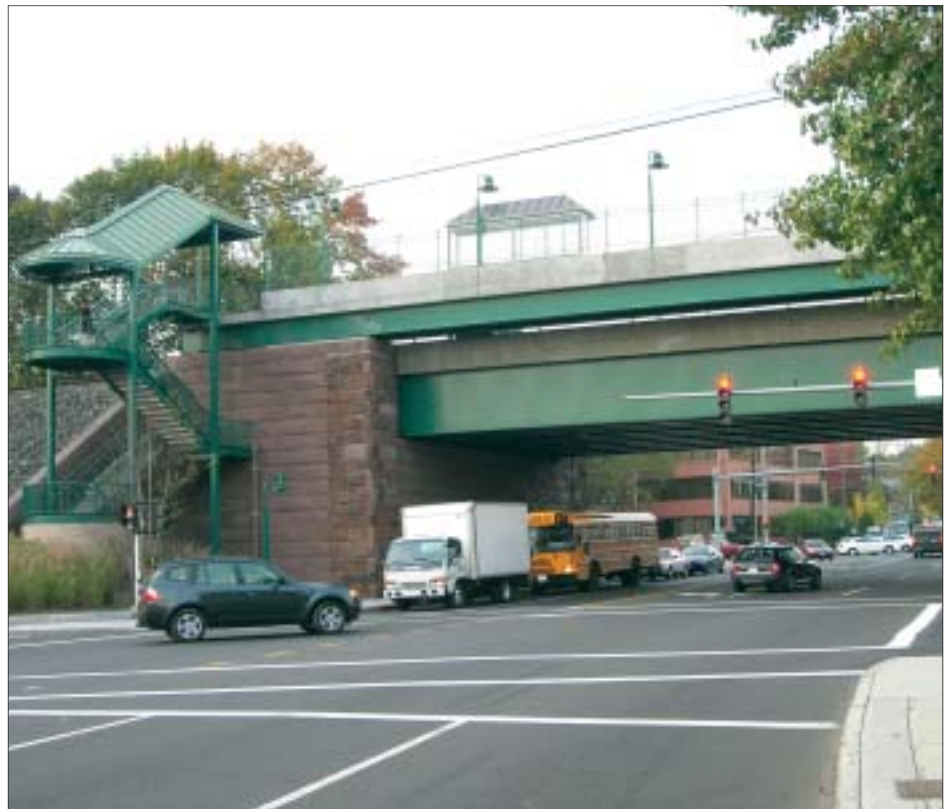
New Arch Street Bridge with pedestrian platform.
