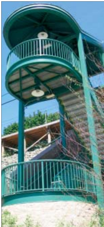
New stair structure.
