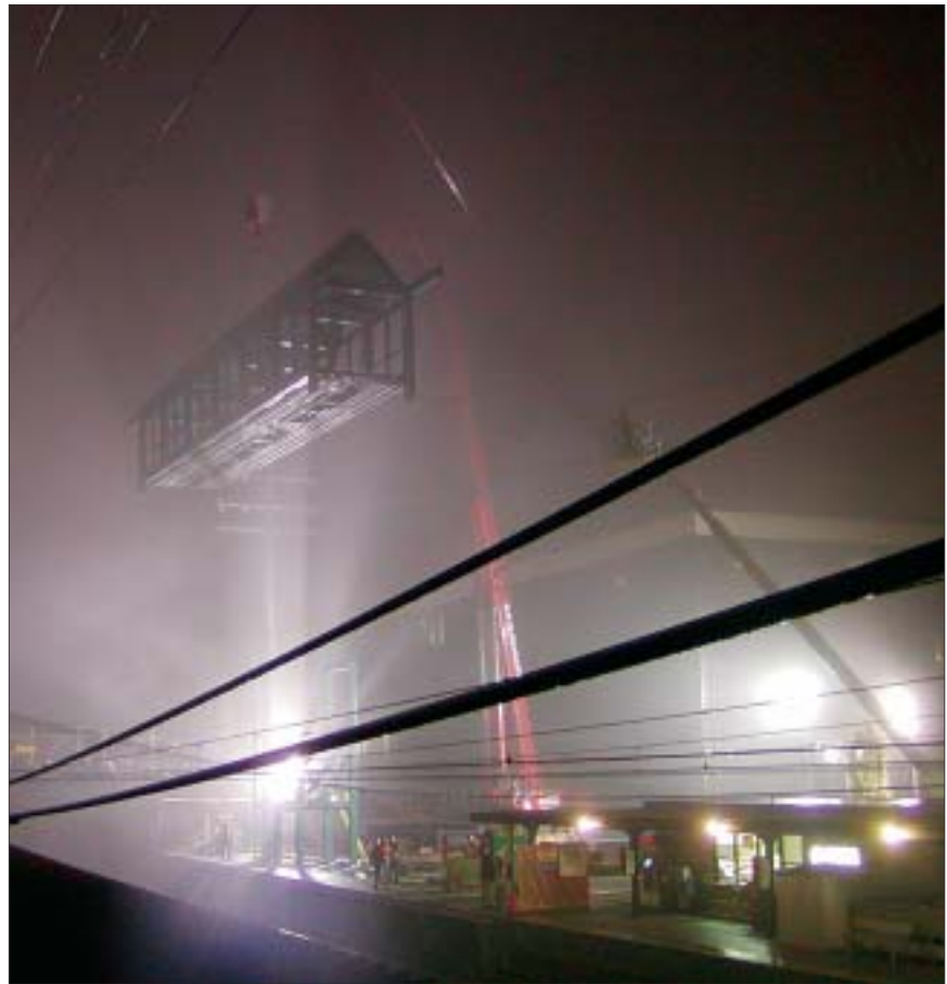
Erection of the pedestrian bridge.
