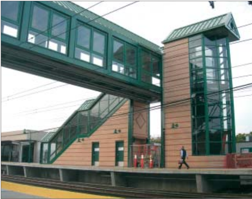
New pedestrian bridge with elevator tower.
