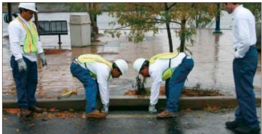
...placed the filter, and put the grate back in place, completing the installation.
