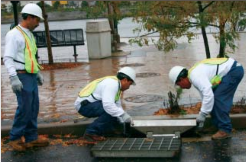
In less than 45 minutes, these installers lifted the grate,...
