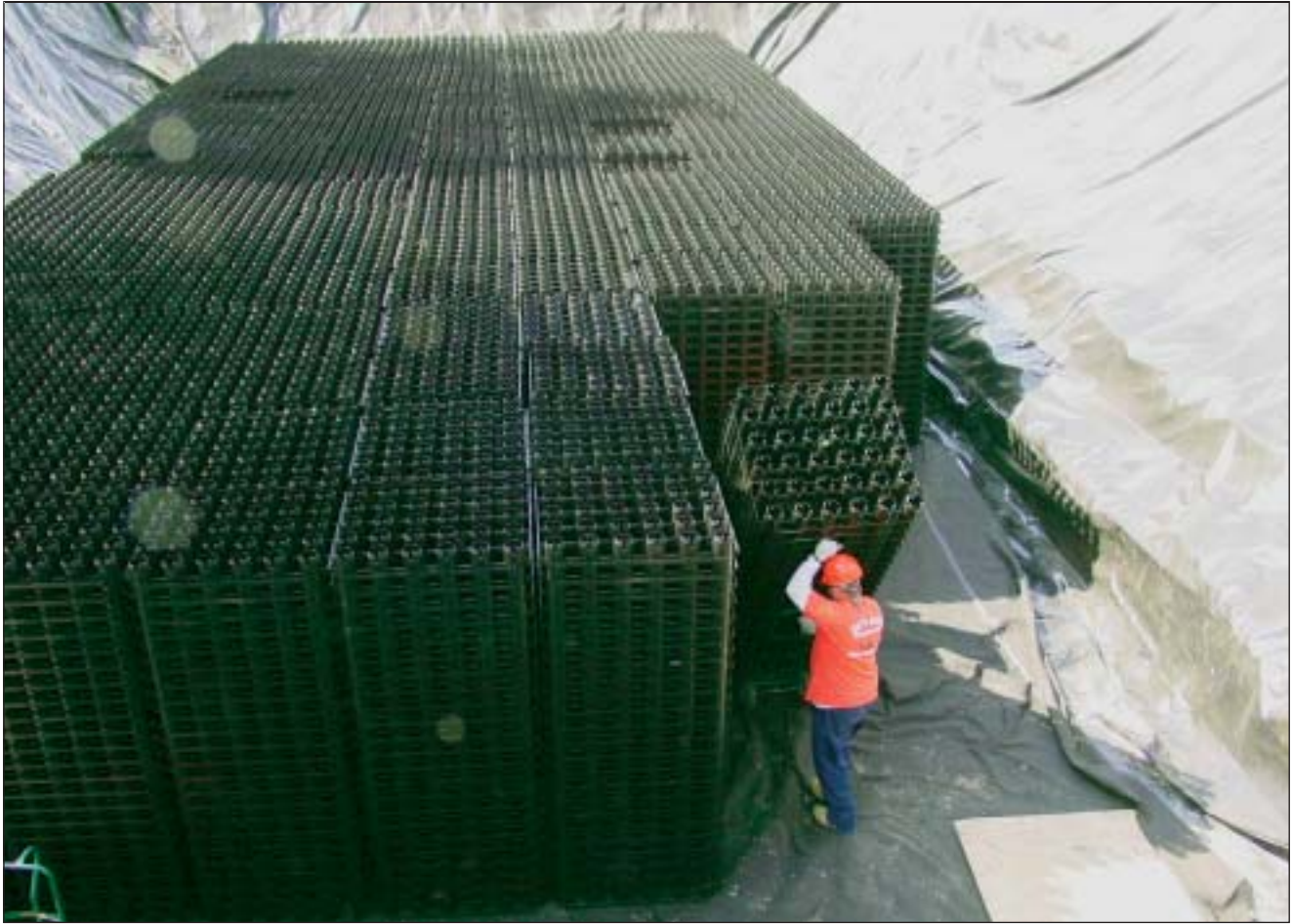
Units are so lightweight they can be moved into position with a hand truck. Made of polypropylene, they can be stacked up to 2.5 meters high (about 8 ft). Properly installed, they create a storage vault with 94 percent void space and a load-bearing strength rated at H-20.
