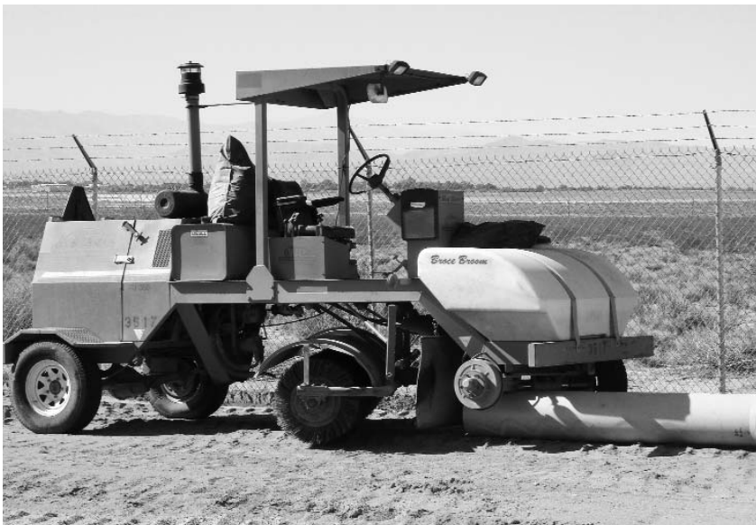
The PVC pipe is incredibly strong. When a piece of heavy machinery blew a tire, a section of the pipe was used to prop up the vehicle until it could be repaired.
