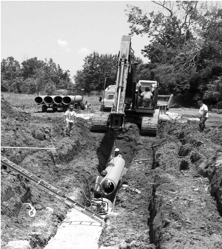
Because SaniTite HP from ADS is lighter than solid wall PVC or concrete pipe, contractors can lay 20-ft sticks at a time.
