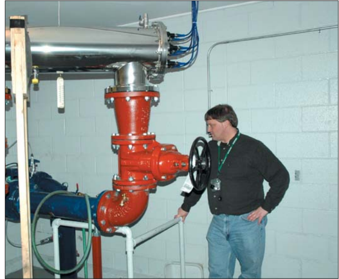
Wedeco UV Reactor—supplied by ITT Water & Wastewater—undergoes inspection.
