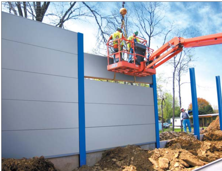
Cost of the CENTRIA composite sound barriers is about one-third that of precast concrete.
