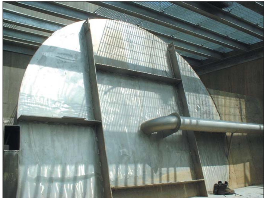
The Hydrobrake® Flow Control is a self-activating vortex flow control device that harnesses the energy inherent in the flow field. They have no moving parts and no external energy requirements. With clear openings up to 600 percent, the risk of blockage is minimized. In addition, the head/discharge characteristics with high flush and kick-back flow points, reduce storage volume requirements, lowering project costs.
