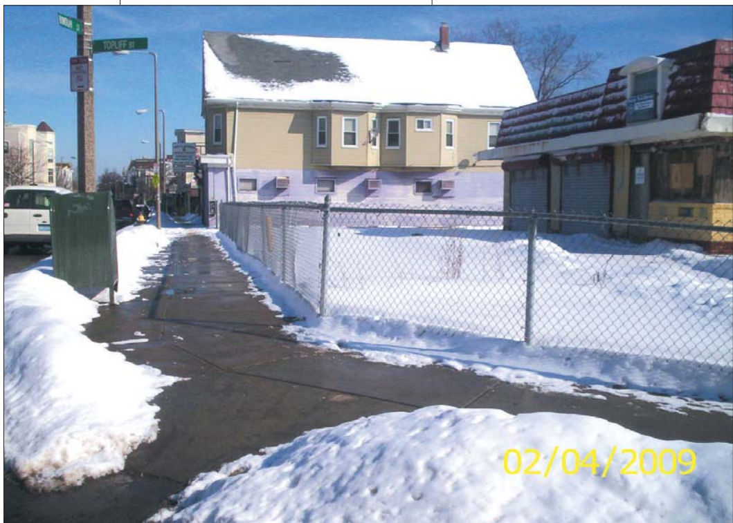
The property was used as a gasoline filling station from about 1931 through 1990. The building has since been standing vacant. With this type of land use, the site has a long history of underground petroleum storage. Abandoned gasoline underground storage tanks exist on the site, as well as contamination in the soil and groundwater. The types of contaminants found at this site are generally consistent with those of petroleum contamination from gasoline products and lubrication oils.
