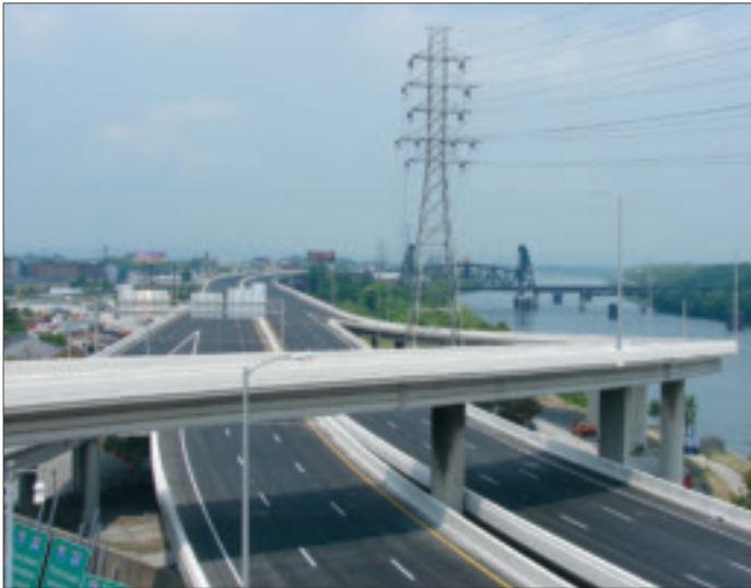
The $53-million Riverside Expressway (I-64) project included the replacement of 132 expansion joints for 14 bridges plus structural steel repairs and facility upgrades.
