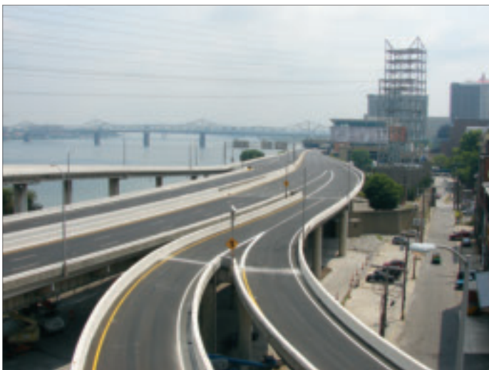
A one-step waterproofing/wearing course system—Rosphalt 50—was used for the new riding surface so the work could be completed during the time allotted.
