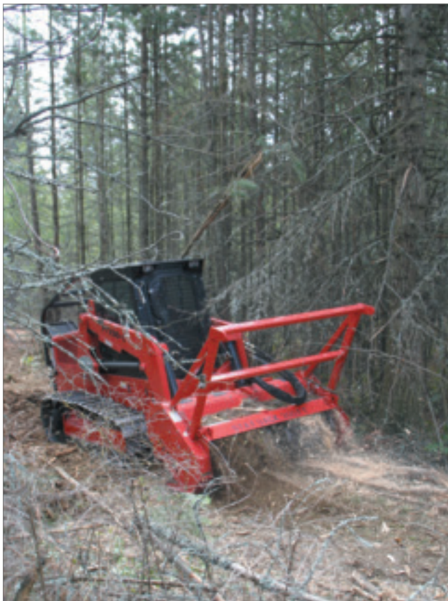
A Fecon FTX90 mulcher shreds underbrush and standing trees to six in. in diameter, making quick work of trail grooming projects.
