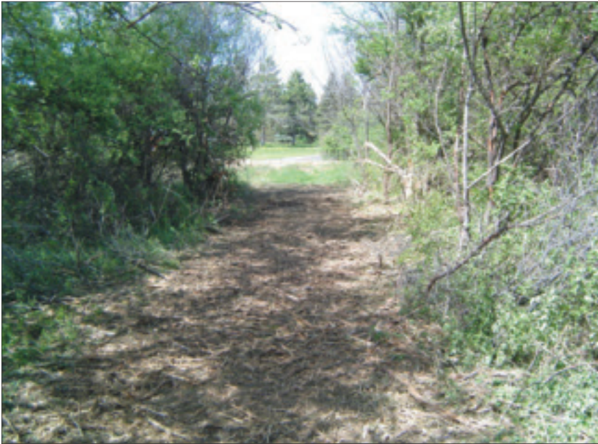
A trail cut through fairly dense underbrush with a single pass of a mechanical mulcher.
