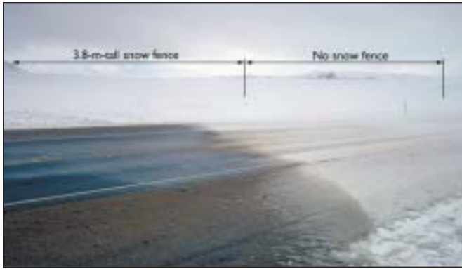
Figure 1. Transition from frozen slush to wet pavement corresponds to the beginning of the area protected by a 12.4-ft snow fence located about 500 ft upwind.
