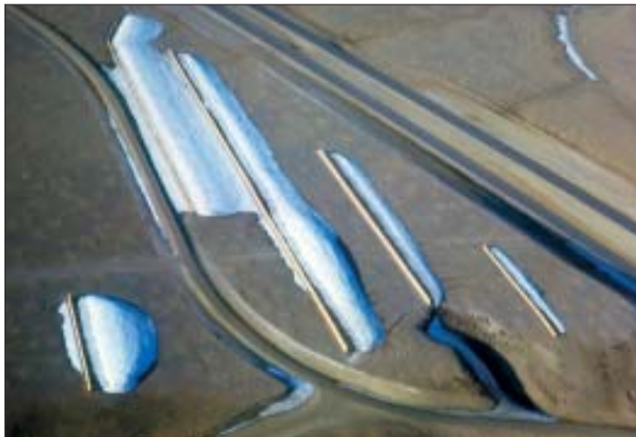
Aerial view shows the snow fence system at Wyoming I-80 Mile 280.8.
