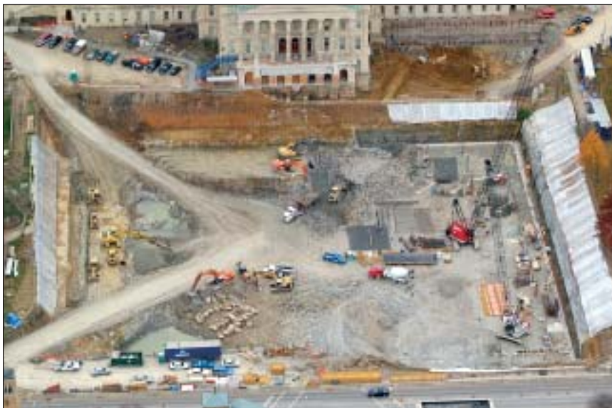
Aerial view of parking garage and northwest mechanical vault construction.
