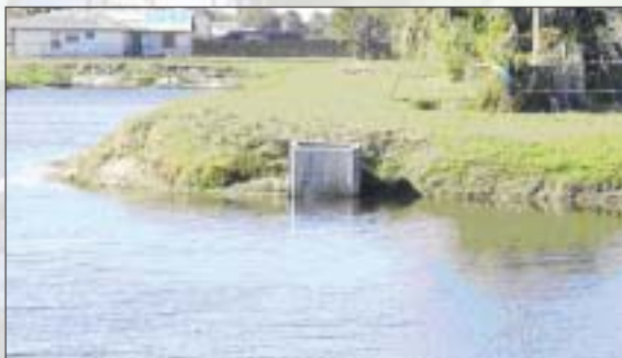
Because PVC is inexpensive, non-corrosive, and durable, it is a good choice for barriers at control structures.
