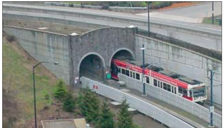
Trimet's Westside Metropolitan Area Express (MAX) line has a portion of its tracks constructed in a tunnel through Portland's West Hills neighborhood. The agency has adopted numerous new safety measures.
