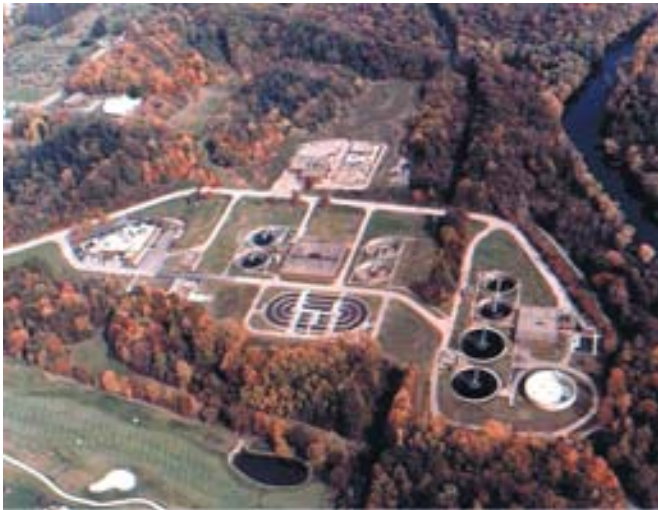
Ten wastewater treatment plants are operated by the Summit County (OH) Department of Environmental Services.
