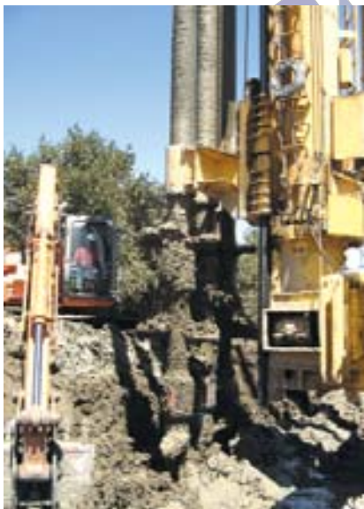
A triple auger DSM rig installs a cutoff wall.
