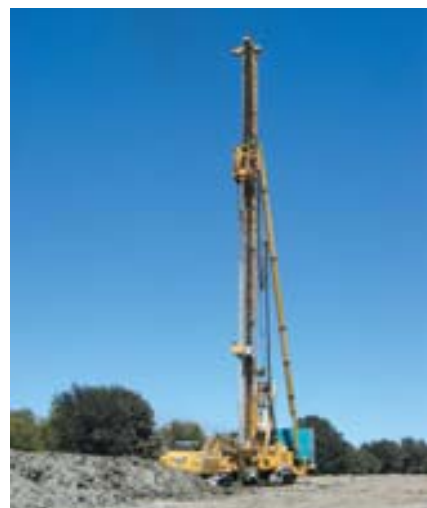
DSM rig with an 80-ft mast.
