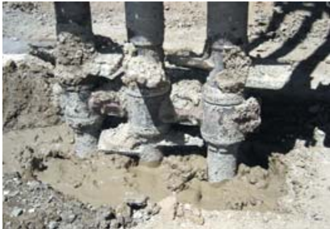
Mixing of the soil-cement-bentonite cutoff wall.
