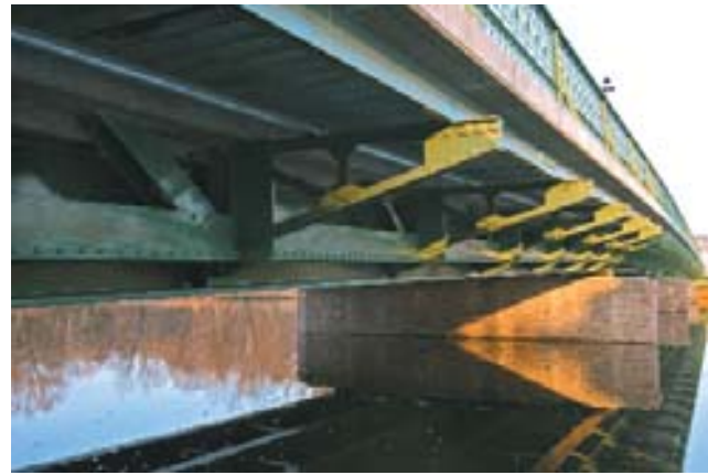
At left is a view of the sidewalk brackets and lower portion of the truss on the original Hillery Street Bridge. At right, a view of the new cantilevered sidewalk brackets from the underside of the replacement bridge.
