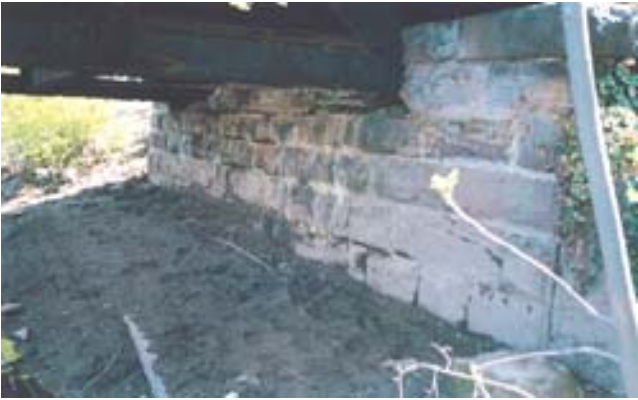
Once both abutments were relaced with new reinforced concrete abutments founded on spread footings, stone facing was attached that replicated the general color and appearance of the original stone.
