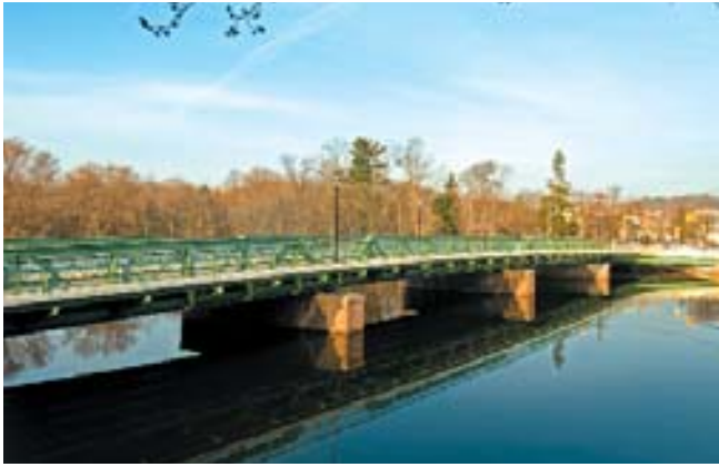
The new Hillery Street Bridge replaces the original, built in 1898. The original was a four-span, simply supported, riveted Pratt Pony Truss carrying one lane of traffic in each direction across the Passaic River in northern New Jersey.
