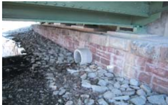
Once both abutments were relaced with new reinforced concrete abutments founded on spread footings, stone facing was attached that replicated the general color and appearance of the original stone.
