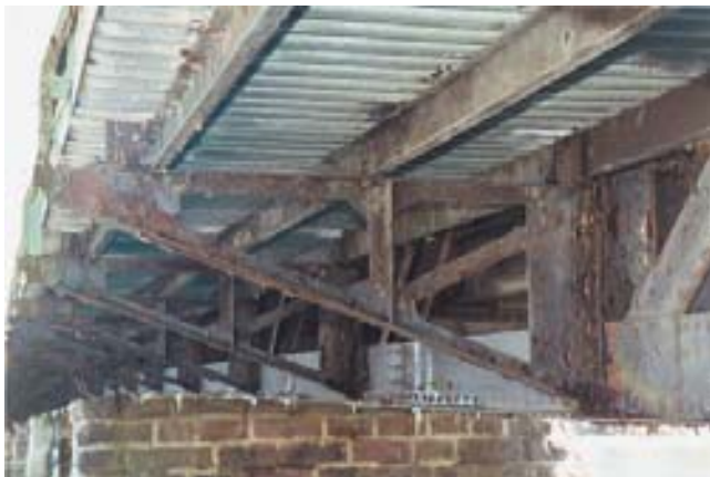
At left is a view of the sidewalk brackets and lower portion of the truss on the original Hillery Street Bridge. At right, a view of the new cantilevered sidewalk brackets from the underside of the replacement bridge.
