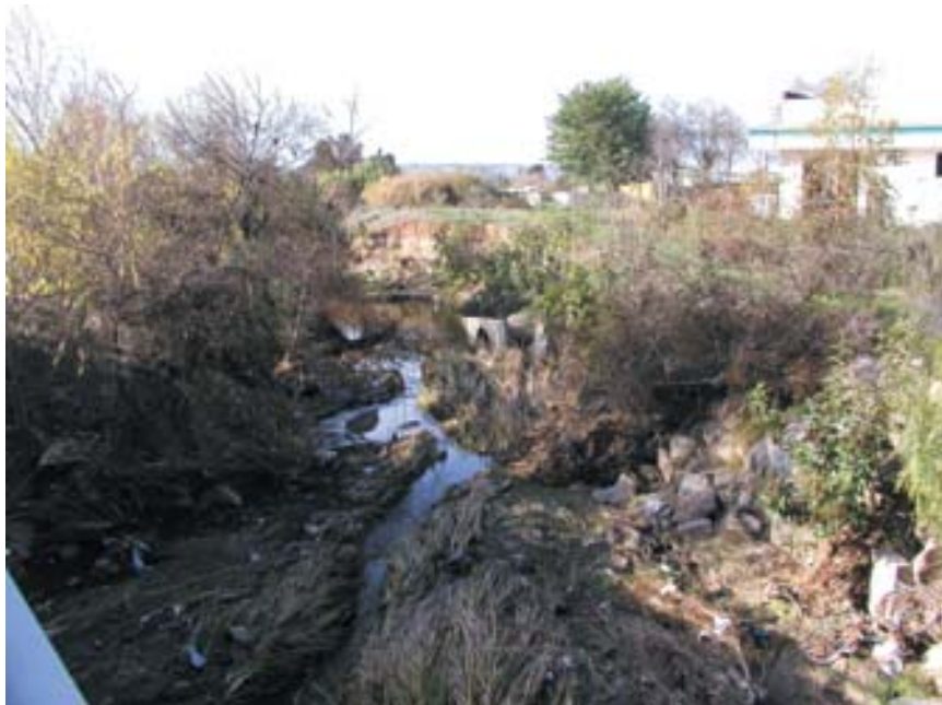
Before the Forester Creek Improvement Project began, the creek was strewn with debris, overgrown with invasive vegetation, and attracted transients. Photo credit: PBS&J
