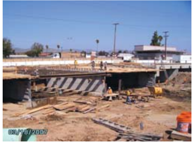
At left, to contain a 100-year flood event, Forester Creek was widened by up to 200 ft in some areas, roughly three times its original size. On the right, to accommodate the widening of Forester Creek, the Mission Gorge Road Bridge had to be doubled in length. Mission Gorge Road, a major arterial, is used by 50,000 vehicles daily. Photo credit: PBS&J
