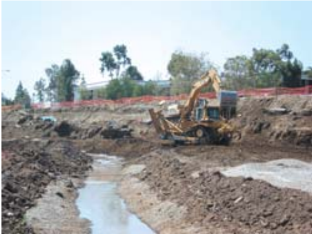
At left, to contain a 100-year flood event, Forester Creek was widened by up to 200 ft in some areas, roughly three times its original size. On the right, to accommodate the widening of Forester Creek, the Mission Gorge Road Bridge had to be doubled in length. Mission Gorge Road, a major arterial, is used by 50,000 vehicles daily. Photo credit: PBS&J
