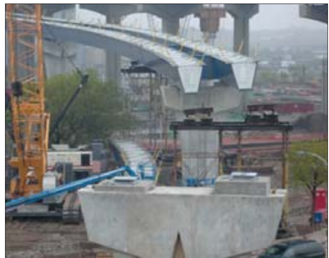
The trapezoidal steel box ramps are highly resistant to cracking.
