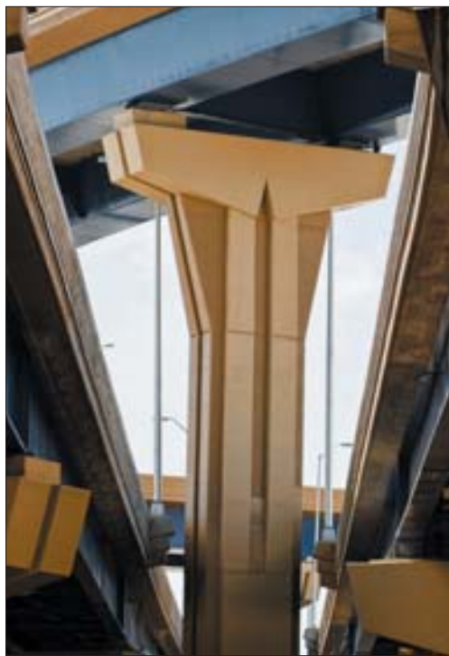
The new design combined steel plate I-girders, steel box girders, and prestressed concrete beams. Photo by Richard Publitz.
