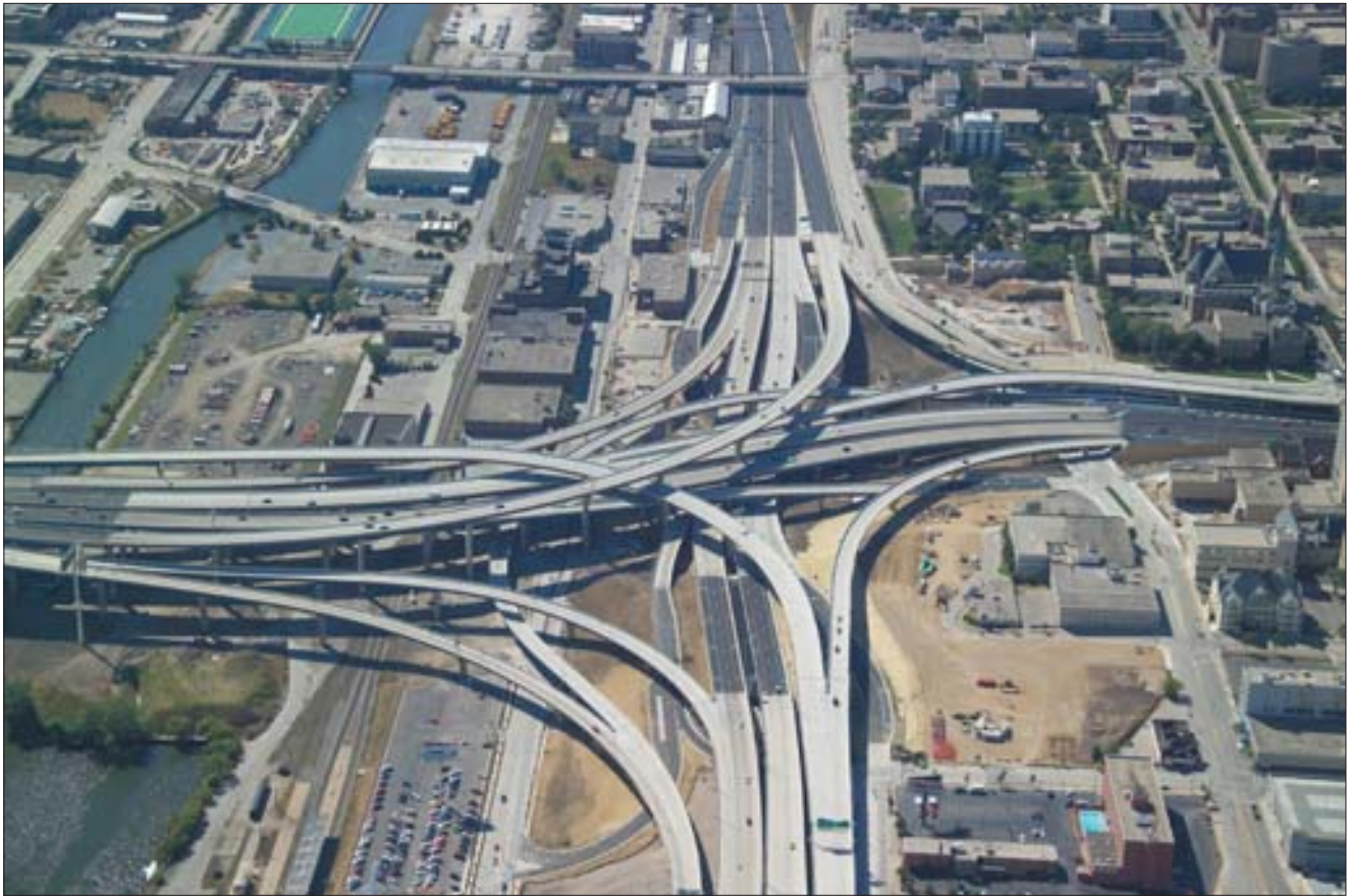
Aerial view of the Marquette Interchange construction project upon completion.
