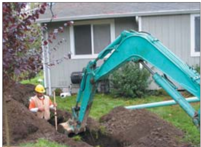
Typical side sewer installation job site.
