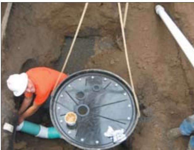
Connecting side sewer to valve pit.
