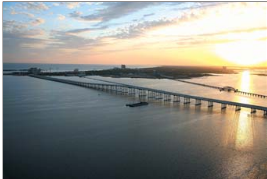
The Biloxi Bay Bridge connects Biloxi on the west with Ocean Springs on the east. Photo by John Thomas Photography.
