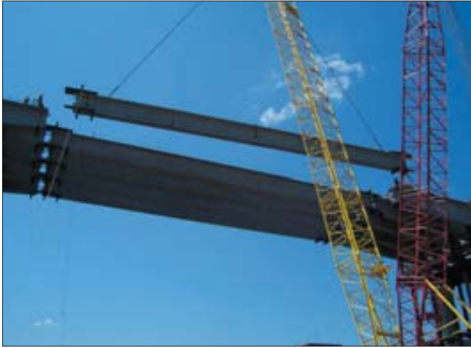
The main navigation span provides 250-ft horizontal clearance and 95-ft vertical clearance.
