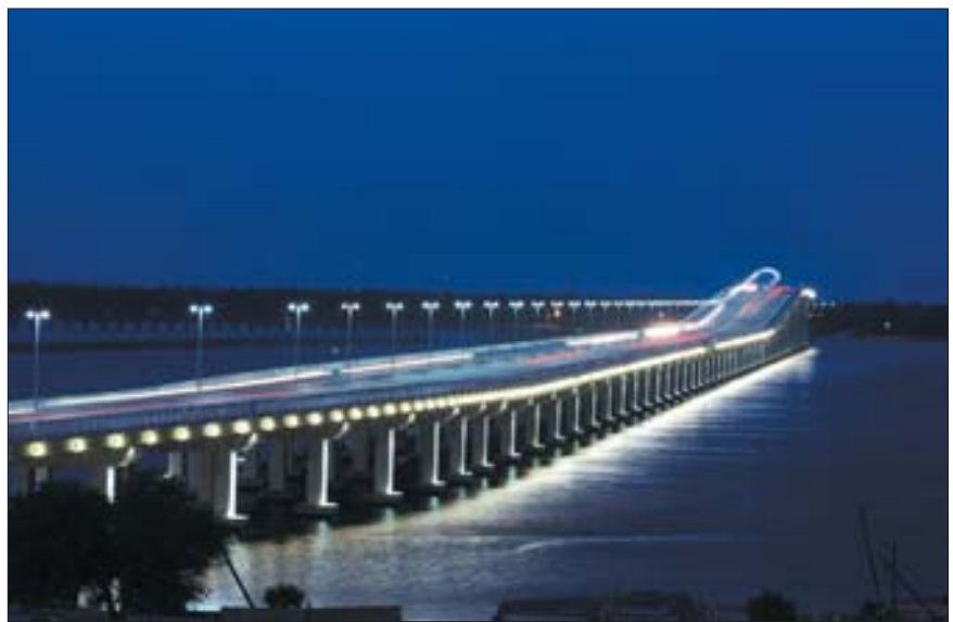
The Biloxi Bay Bridge lighting illuminates both the edge beam and the piers. Photo by John Thomas Photography.
