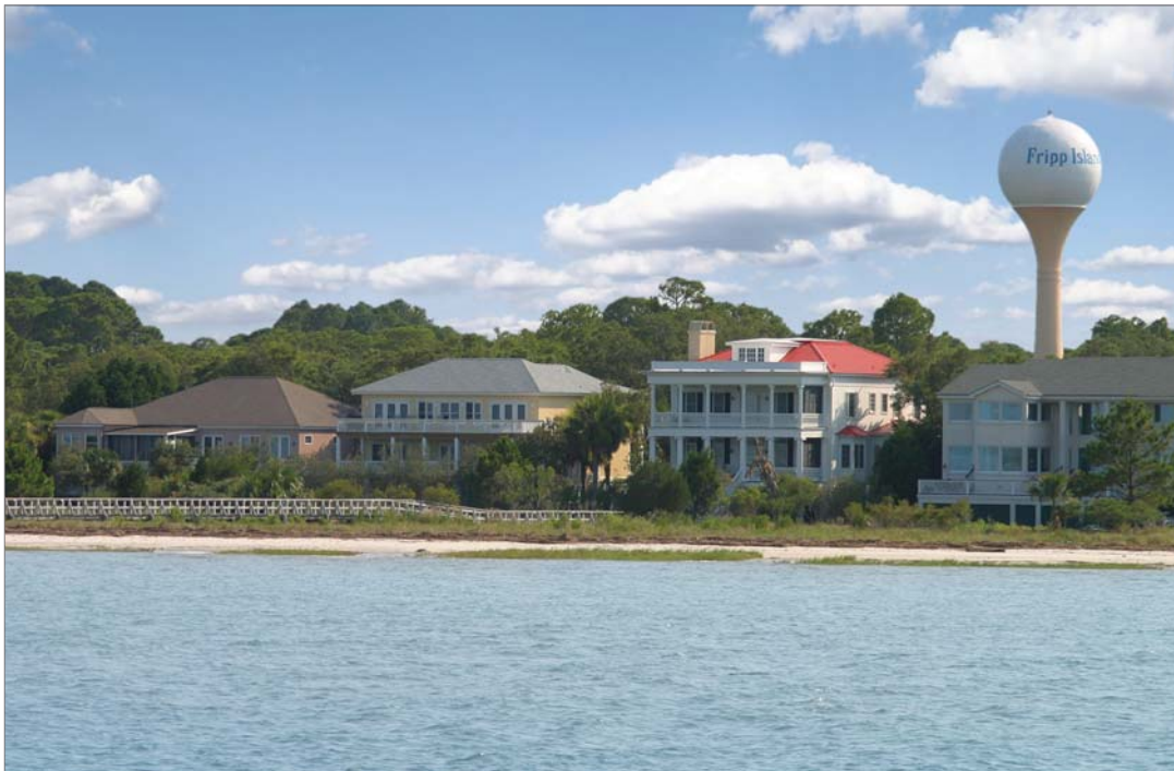
Vacuum sewer technology is a cost-effective solution for communities with flat topography, sandy soil, and a high water table, like Fripp Island, SC.
