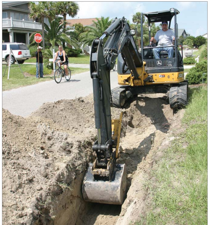
Vacuum sewers are typically buried in shallow trenches, so contractors can use smaller excavation equipment and there is less soil displacement, allowing streets to remain open.
