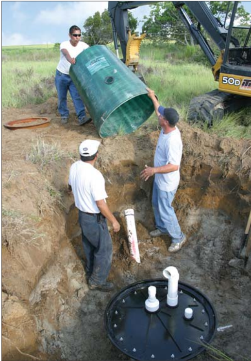
AIRVAC components are lightweight yet extremely durable; workmen can install most of the components by hand.
