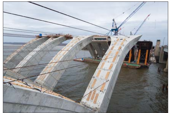
About $1 million in construction value is put in place daily at the Woodrow Wilson Bridge project. Photo by David Sailors.
