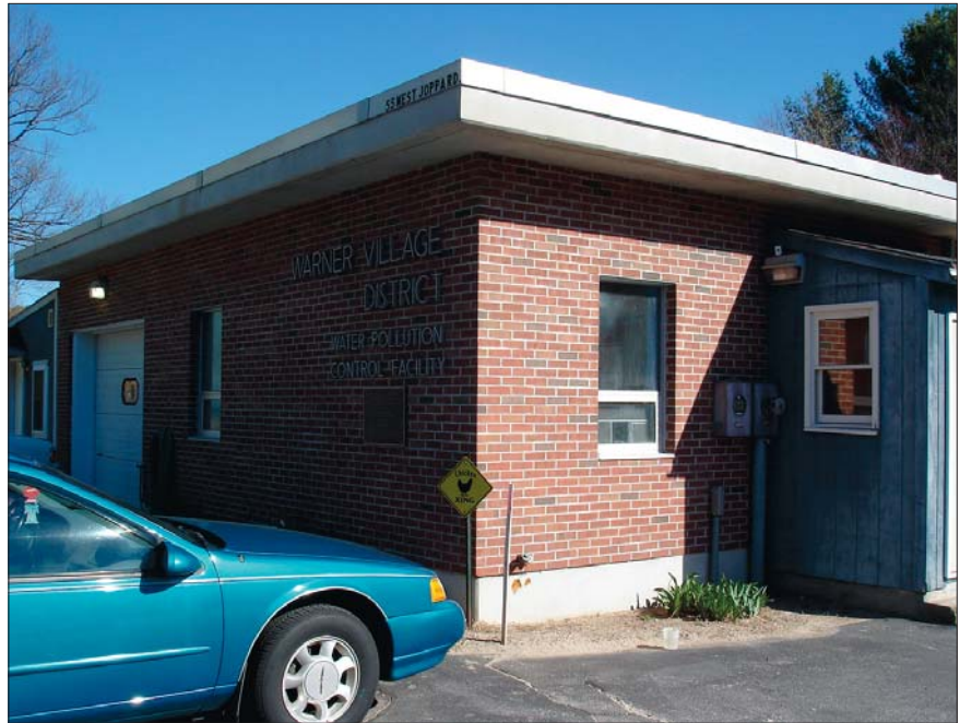
The Warner Village Water District’s award winning wastewater treatment plant came on line in 1976.
