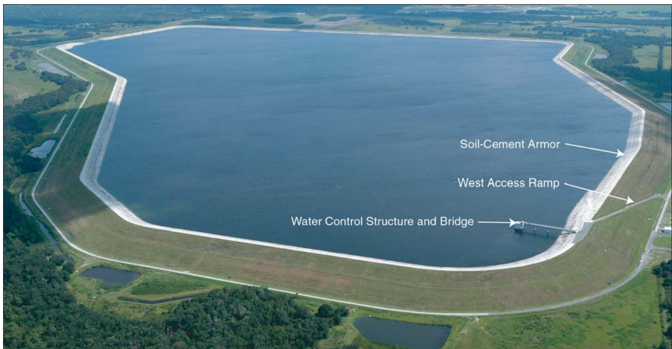
Aerial view of Tampa Bay Reservoir during initial filling in August 2005.
