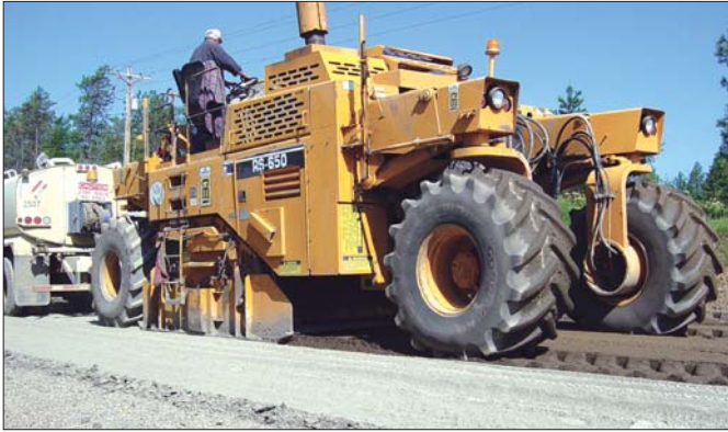
... the placement of cement ...
