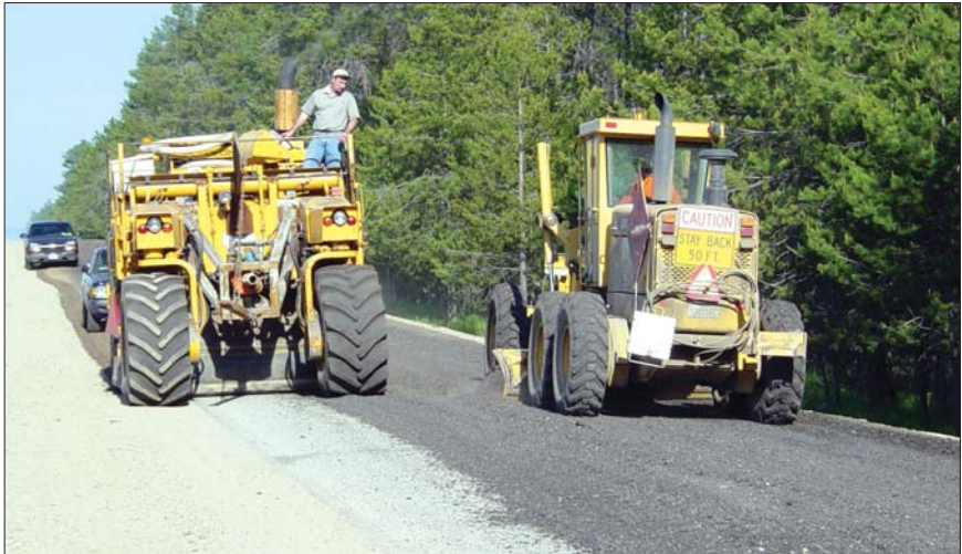
First, Spokane County pulverizes the road ...
