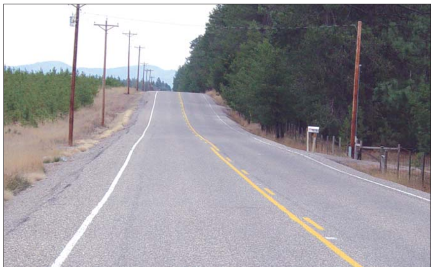
... finished with a layer of crushed stone and bituminous surface treatment.
