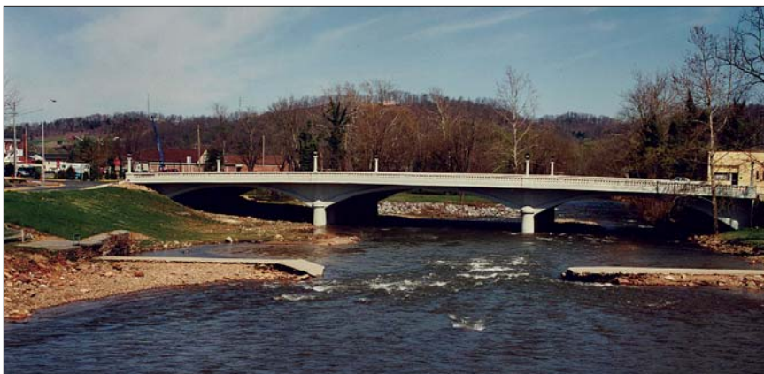
Elk Avenue/Doe River Bridge Rehabilitation, Elizabethtown, TN. Photo courtesy of Tennessee Department of Transportation
