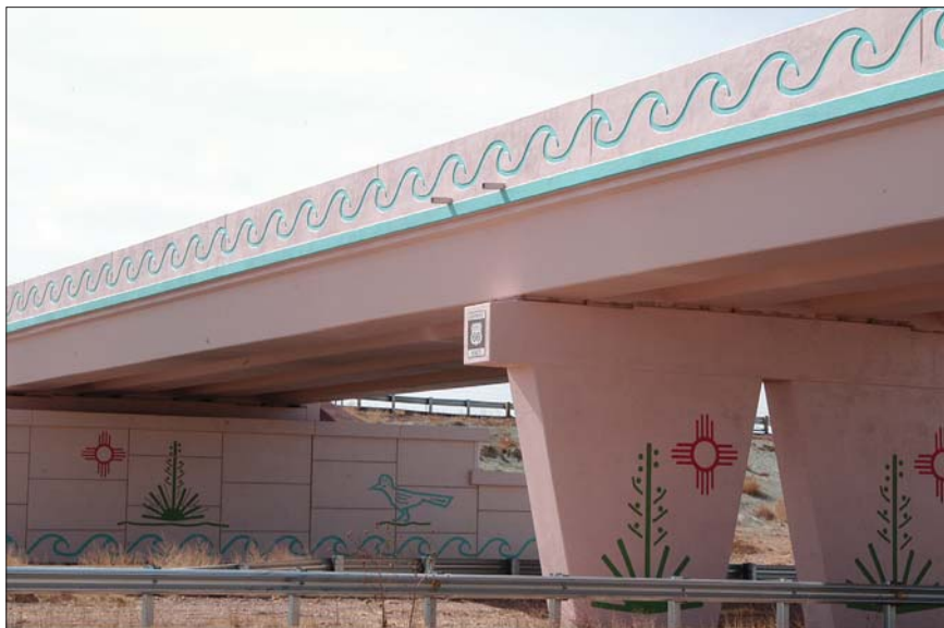
Guadalupe County I-40 Overpass Bridges, Guadalupe County, NM. Photo courtesy of New Mexico Department of Transportation
