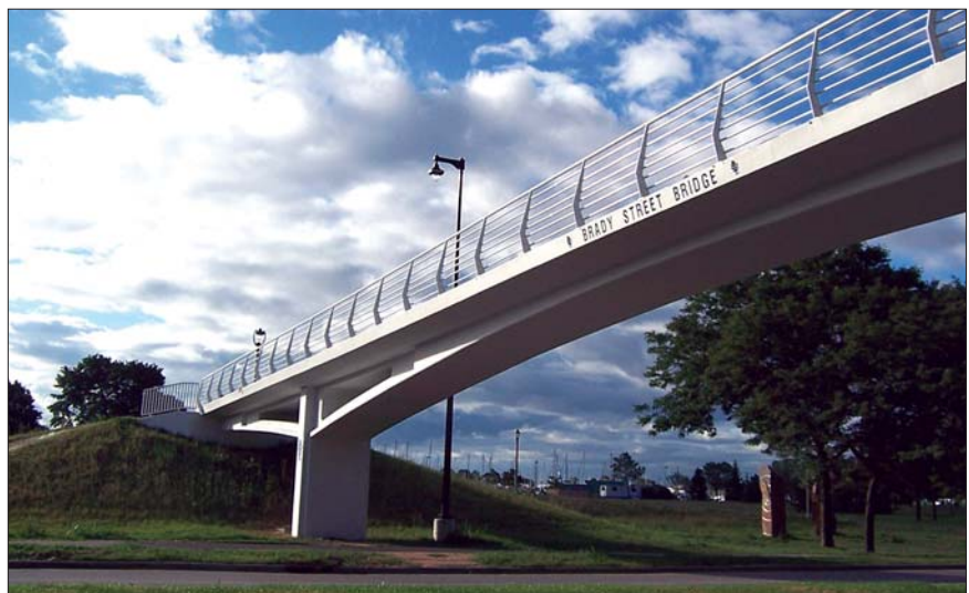
Brady Street Bridge, Milwaukee, WI. Photo courtesy of Bloom Consultants, LLC
