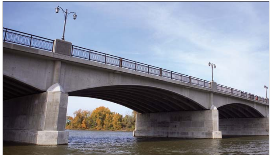
Perry Street Bridge, Napoleon, OH. Photo courtesy of HNTB Corporation
