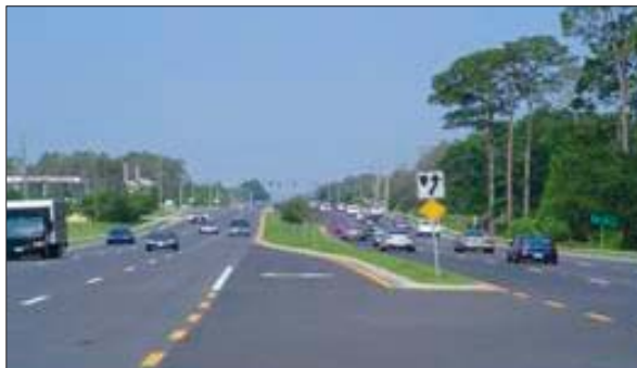
Completed Conroy Windermere Road
