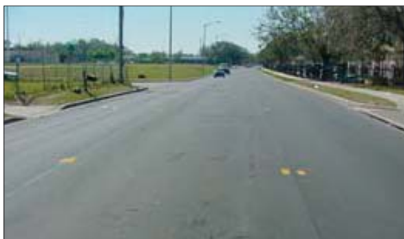
Completed Rio Grande Avenue
