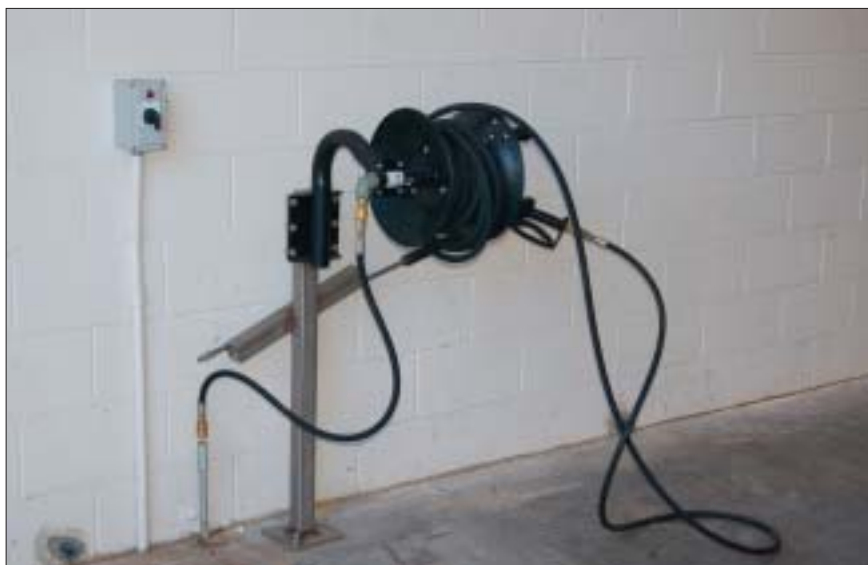
Pressure spray wands operating at 2,000 psi are used to detail engines, wheels, and other parts.
