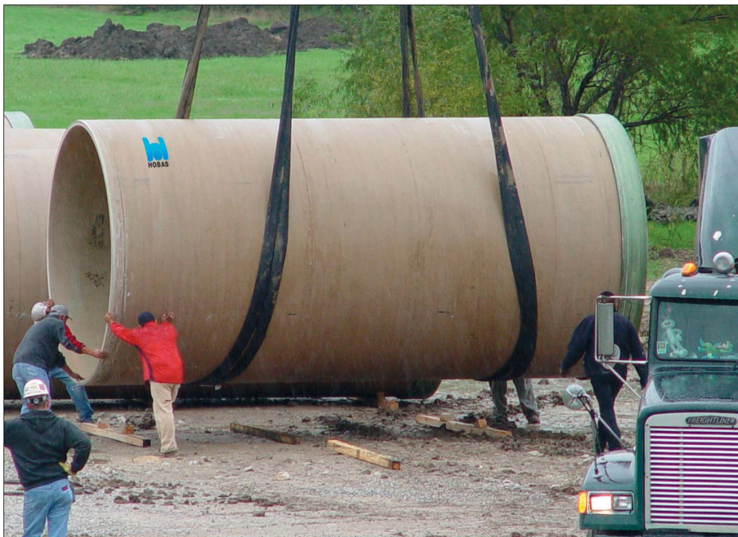
Lightweight CCFRPM pipes are easy to handle at the job site.
