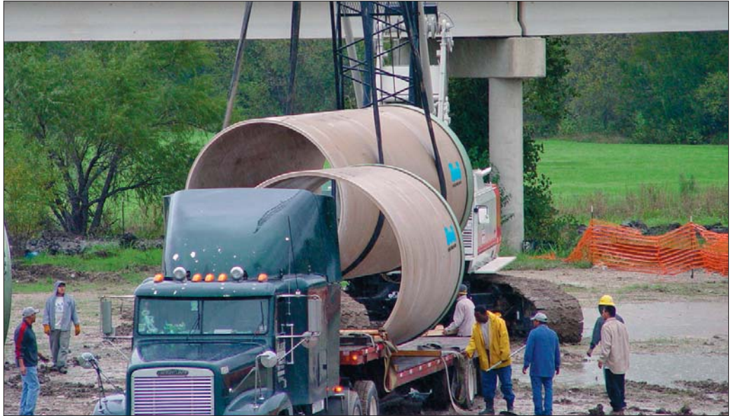
CCFRPM pipes were chosen for the grand Prairie project for long life and corrosion resistance.
