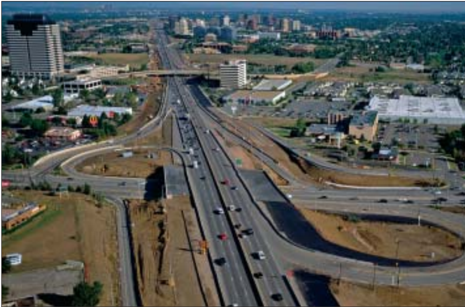
The T-REX Project in Denver is a landmark collaboration between CDOT, RTD, FHWA, and FTA, creating a new streamlined multi-modal approach to project delivery. CDOT, in partnership with the Denver RTD, is reconstructing 16 miles of two interstate highways in the Denver metropolitan area and adding 19 miles of new light rail transit, including 13 stations. The $1.67-billion design-build program is gaining recognition for delivering highway and transit improvements. It was shaped by extensive input from the community, and it is on budget and ahead of the schedule created during the NEPA process.
