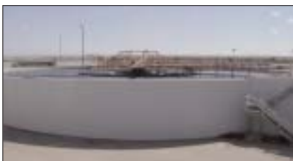
Figure 1. Roberto R. Bustamante Waste Water Treatment Plant.
