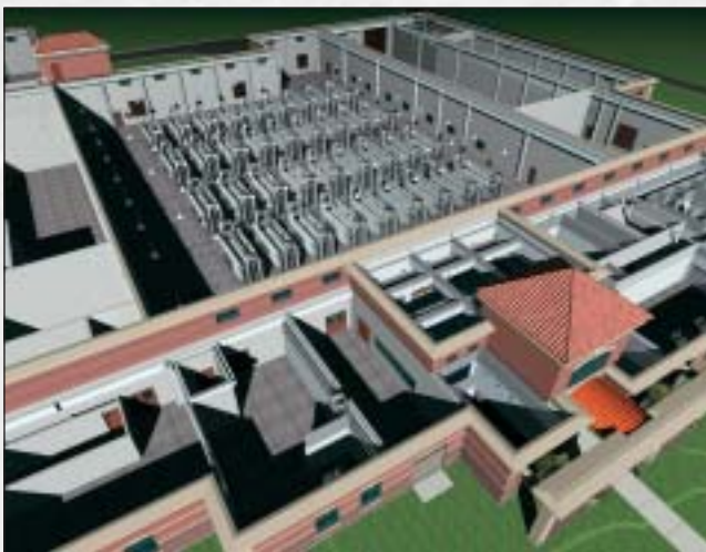
When it begins operation this summer, the MWW's 78-mgd Columbia Heights Membrane Filtration Plant will be the largest membrane facility treating potable water in the world. (Courtesy/Credit: Black & Veatch)
