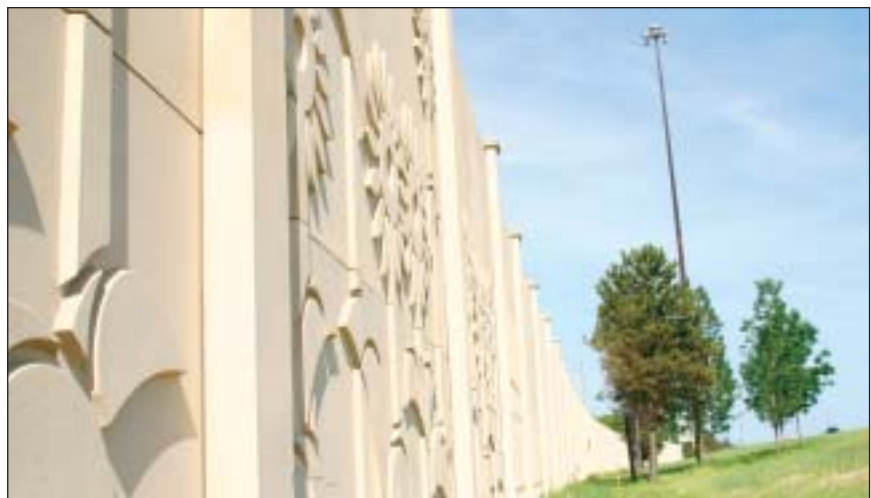
Form meets function on Interstate 94 sound barrier walls in Fargo. Decorative walls feature raised sunflowers, wheat stalks, and trees.
