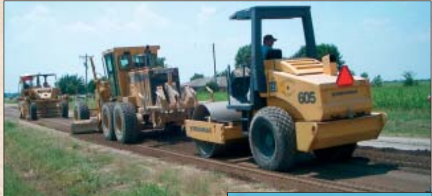
7. Vibratory roller brings up end of processing sequence.
