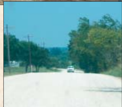
9. Completed test section.
