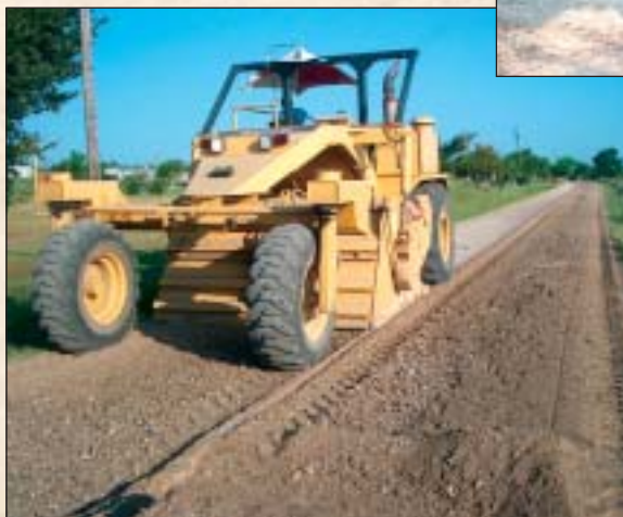
2. Second lane of test section is tilled.
